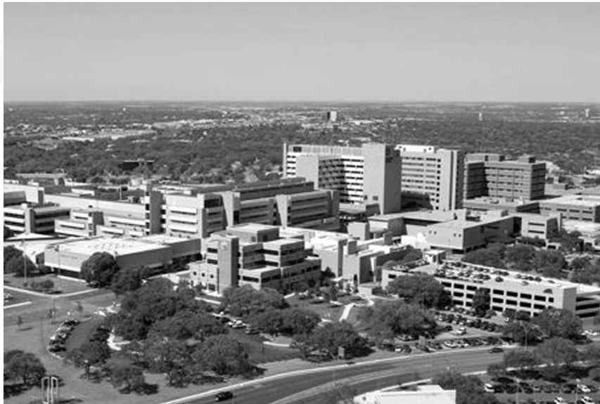
The University of Texas Health Science Center at San Antonio including University Hospital and Audie Murphy VA Hospital
